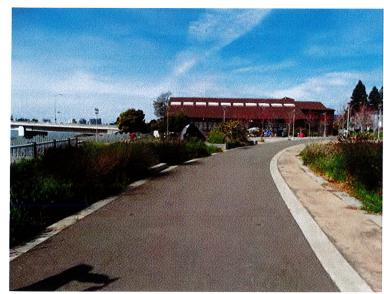
Asphalt path with Concrete Border
