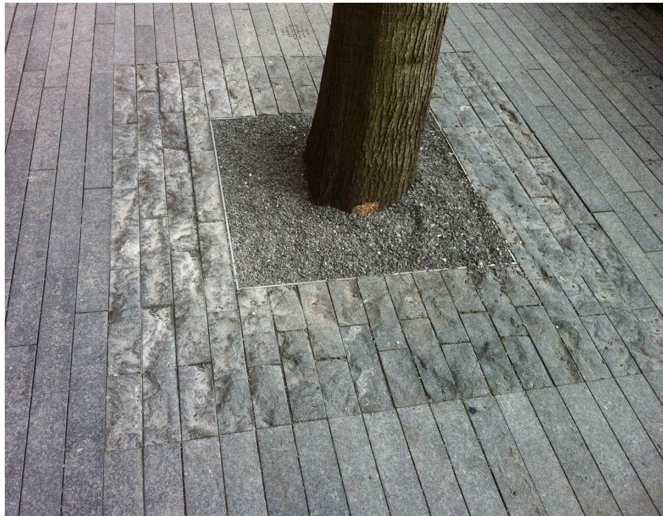
PAVER-COVERED TREE GRATE AT PLANTING TRENCH
