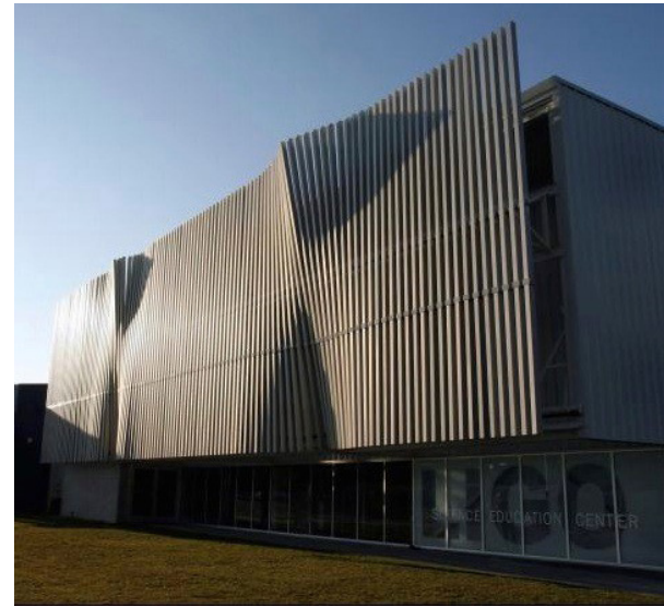
Wind activated aluminum wave wall
