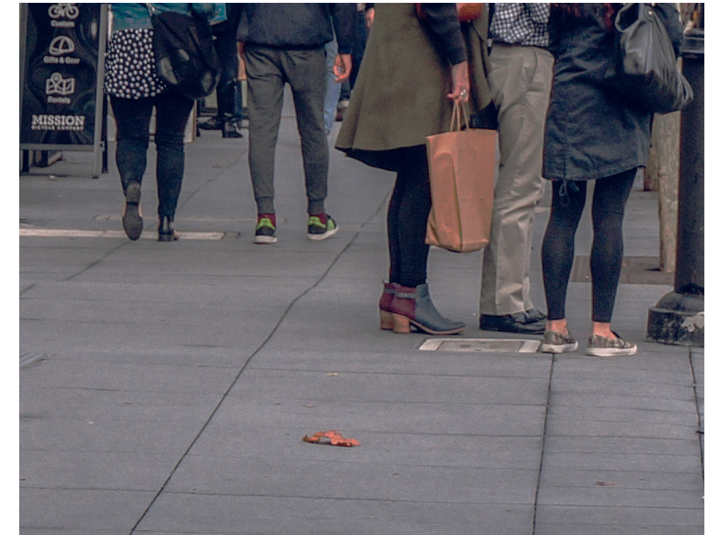
INTEGRAL COLOR CONCRETE SIDEWALK
