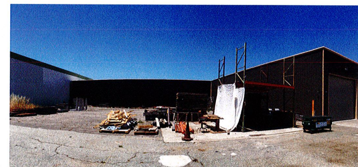
7. (E) LOT LOOKING WEST.
