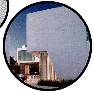
STUCCO OR CEMENT PLASTER WITH COMMON JOINTS
