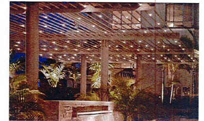
Lights on Trellis
