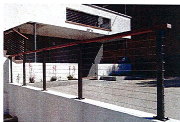
42" HIGH GUARDRAIL ON WALL
