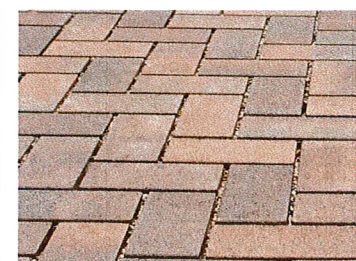
P1. PERMEABLE PAVERS
