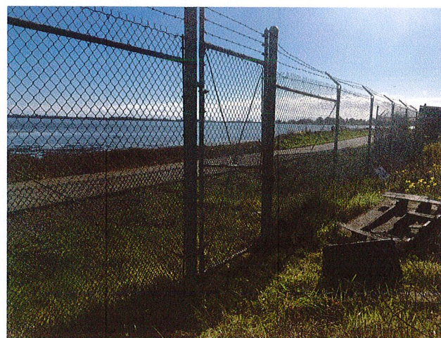
7. SOUTH PROPERTY LINE @ BIKE / PEDESTRIAN TRAIL
