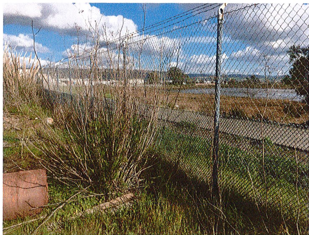
5. SOUTH PROPERTY LINE @ BIKE / PEDESTRIAN TRAIL
