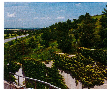
④ RETAINING WALL
