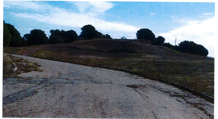
AT EXISTING GATE, LOOKING SOUTHEAST
