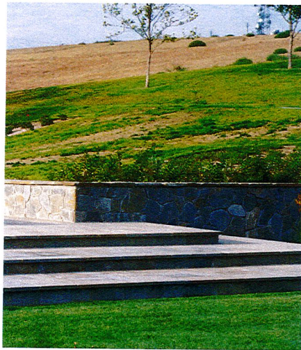
FITTED STONE STEPS
