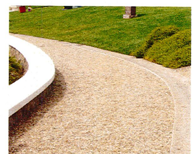
⑤ STABILIZED CRUSHED GRAVEL
