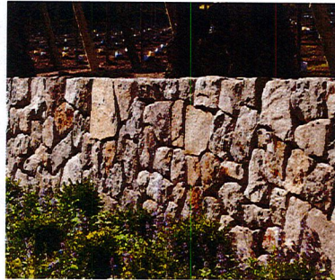
③ STONE RETAINING WALL
