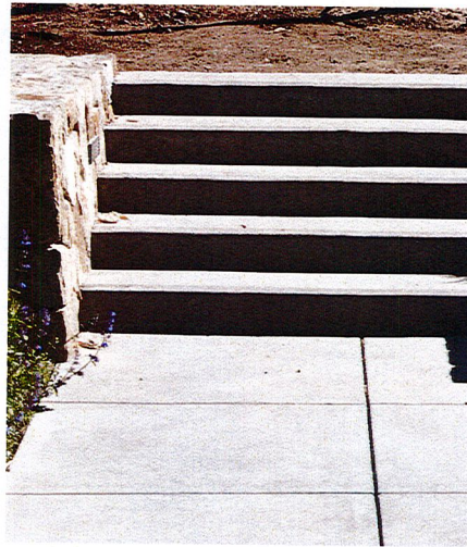
CONCRETE WITH CHEEK WALL
