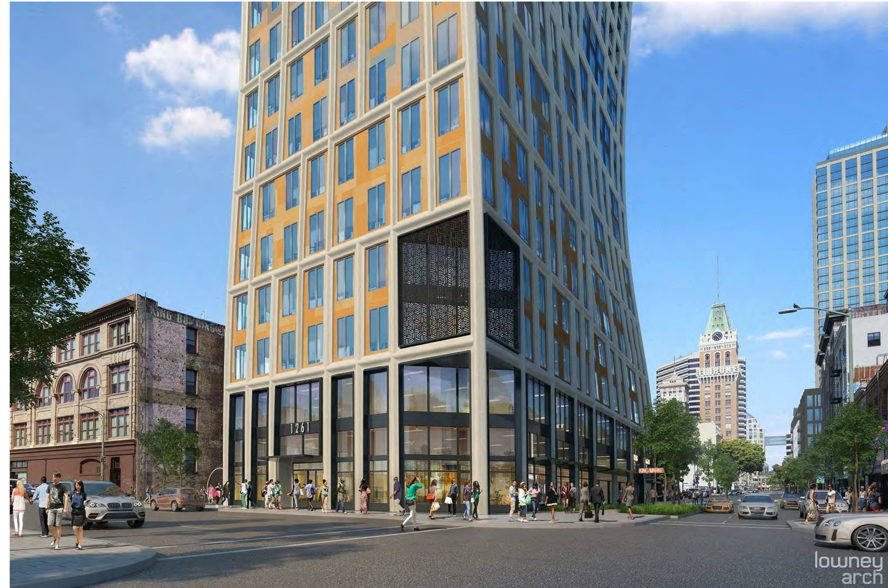
CORNER VIEW AT HARRISON AND 13TH STREET
