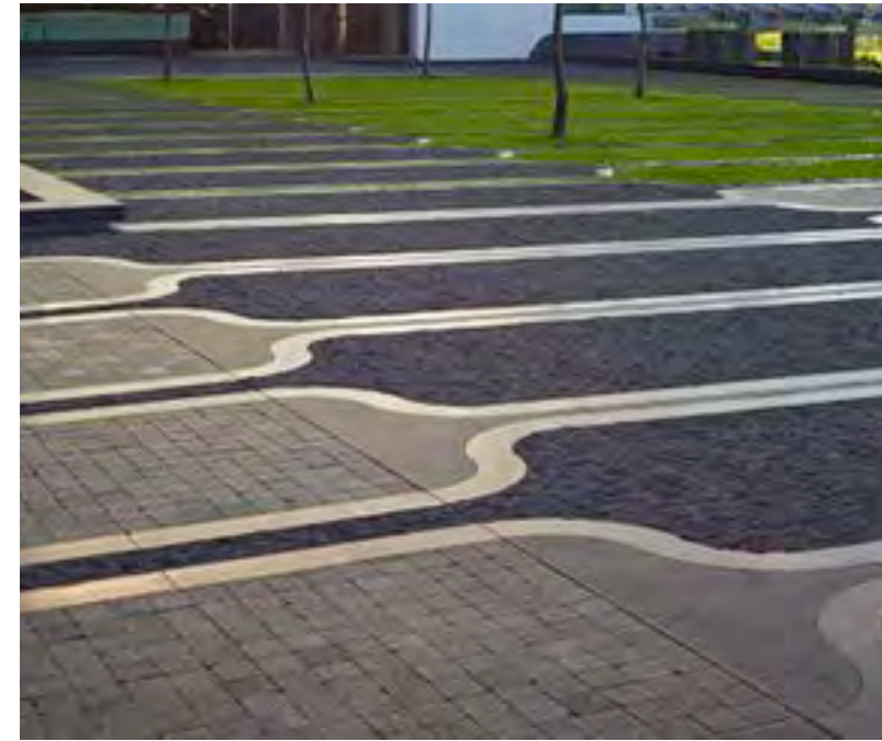
Pattern in special paving Stainless Steel Inlay
