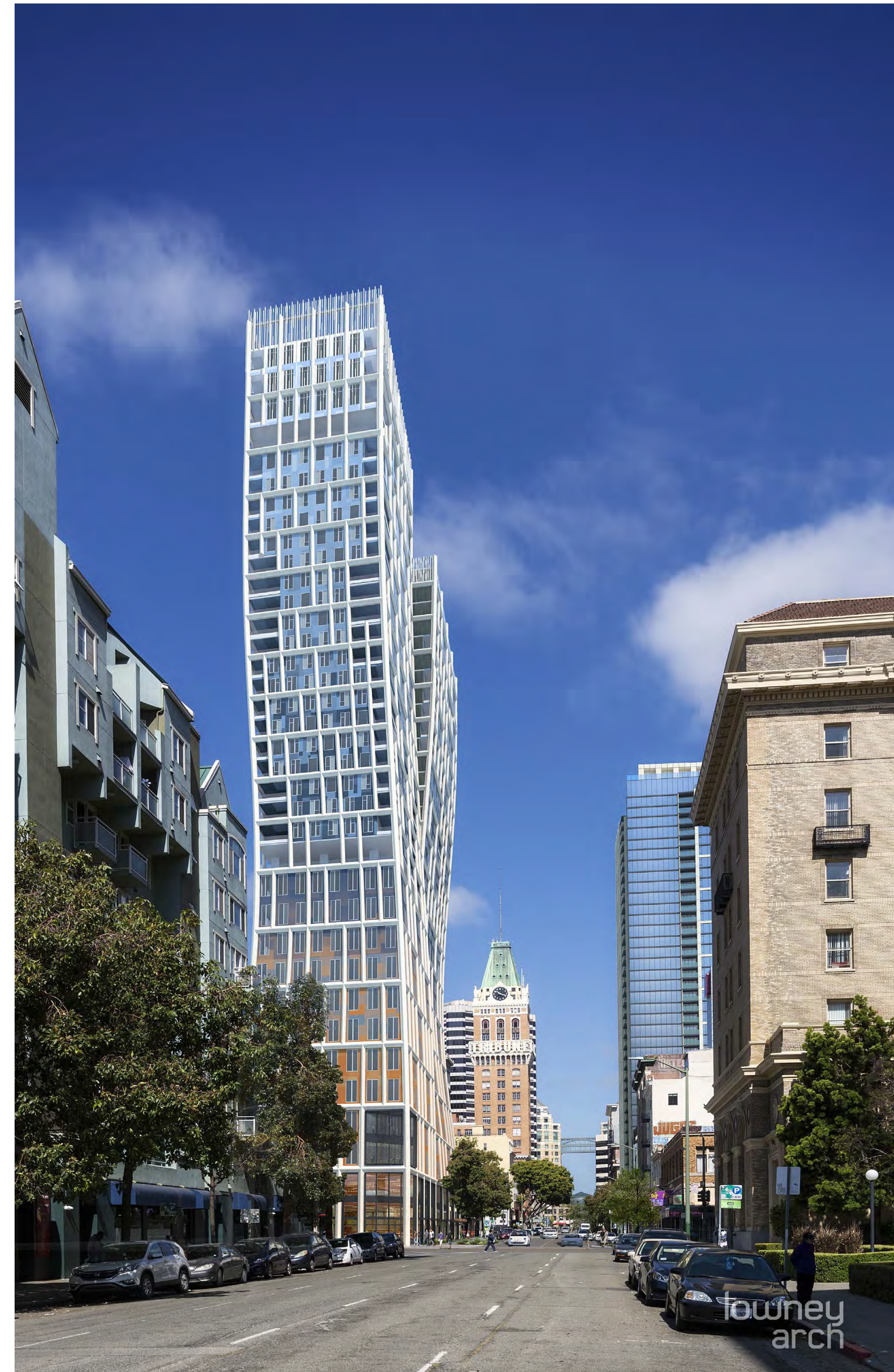
VIEW LOOKING WEST ALONG 13TH STREET
