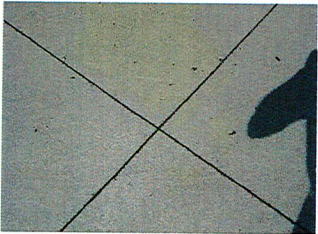
COLORED CONCRETE & SCORING AT ENTRY PLAZAS
