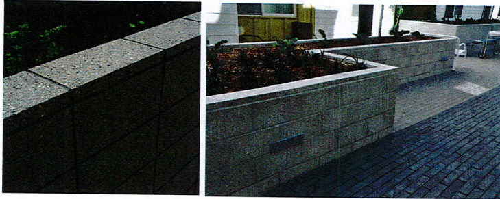
CMU BLOCK WALLS: 6" WIDE WITH GROUND FACE FINISH, DOUBLE WIDE AT SEAT WALL AREAS 16" WIDE
