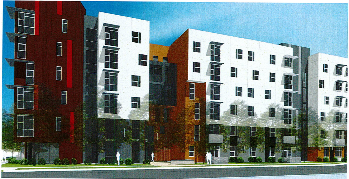
VIEW FACING NORTH ALONG EIGHTH AVENUE
