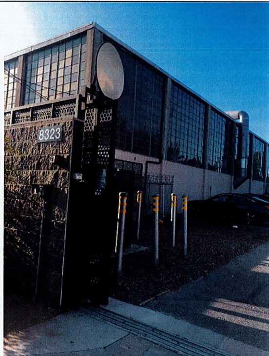
View from LT-1 facing west
