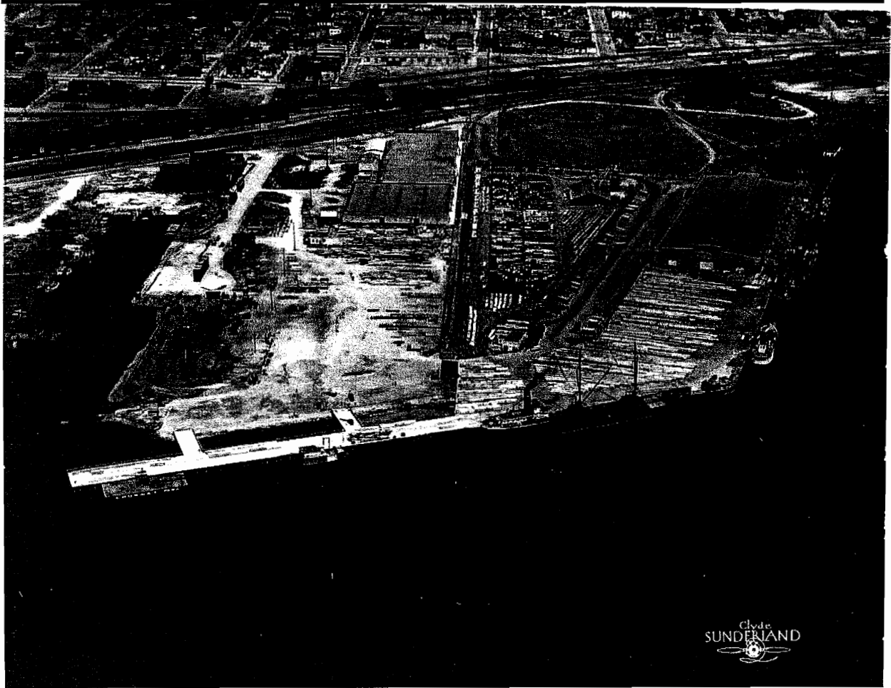
Circa 1930 View of Ninth Avenue Terminal showing transit shed on far right, and steamship docked in front. Quay wall, left of steamship was under construction. (Courtesy Port of Oakland Archives)
