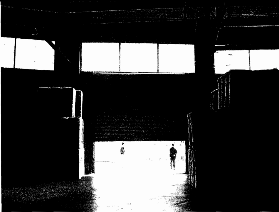
An open bay of the Ninth Avenue Terminal frames a view of Oakland's waterfront
