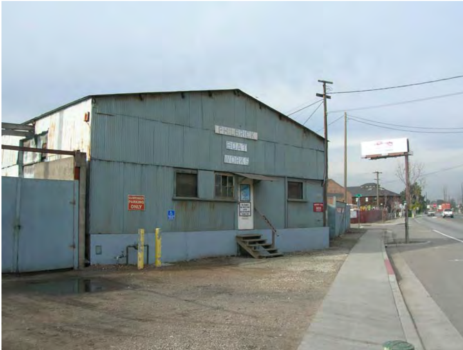
Entrance on Embarcadero ( Carey & Co. December 2005 )
