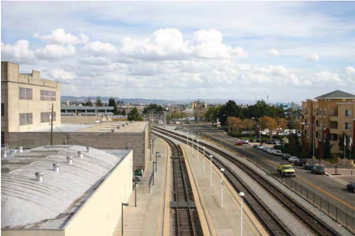
Existing view from Amtrak pedestrian bridge looking southeast (VP3)
