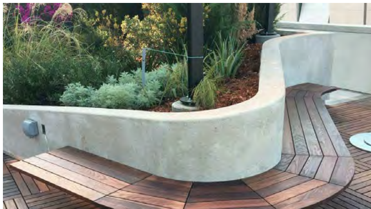
POUR-IN-PLACE CONCRETE WITH SACK FINISH
