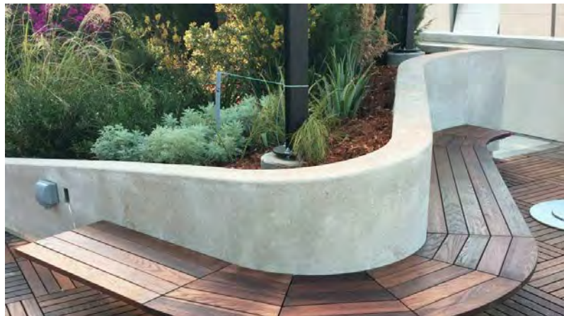
POUR-IN-PLACE CONCRETE WITH SACK FINISH
