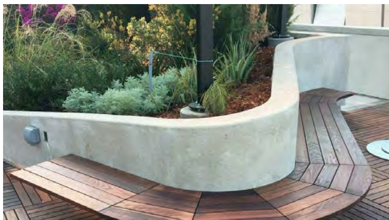
POUR-IN-PLACE CONCRETE WITH SACK FINISH
