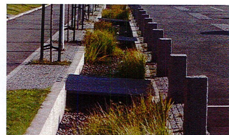
BIORETENTION BASIN w/ METAL GRATE
