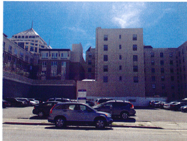
5 SITE, FROM 16TH STREET
