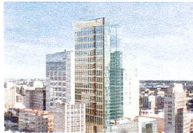
1640 BROADWAY Lennar 380' Under Construction
