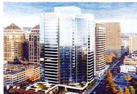
601 CITY CENTER Shorenstein 24 story Under Construction
