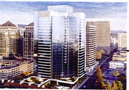
601 CITY CENTER Shorenstein 24 story Under Construction
