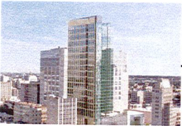
1640 BROADWAY Lennar 380' Under Construction
