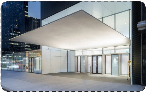
White concrete finish gfrc canopy
