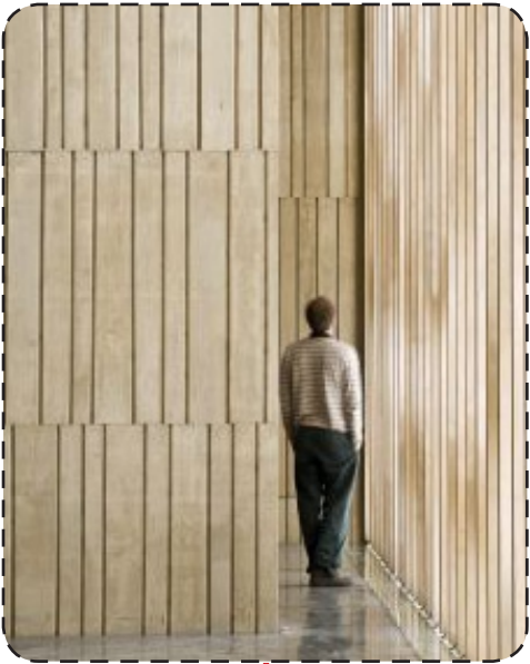
Mechanical area concealed with concrete textured relief
