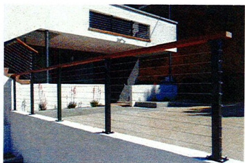
42" HIGH GUARDRAIL ON WALL
