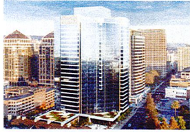
601 CITY CENTER Shorenstein 24 story Under Construction
