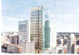
1640 BROADWAY Lennar 380' Under Construction
