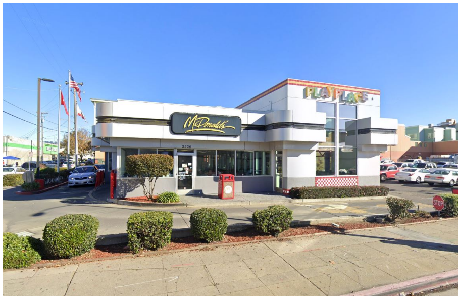
Photo -7 – Front Elevation side of Building
