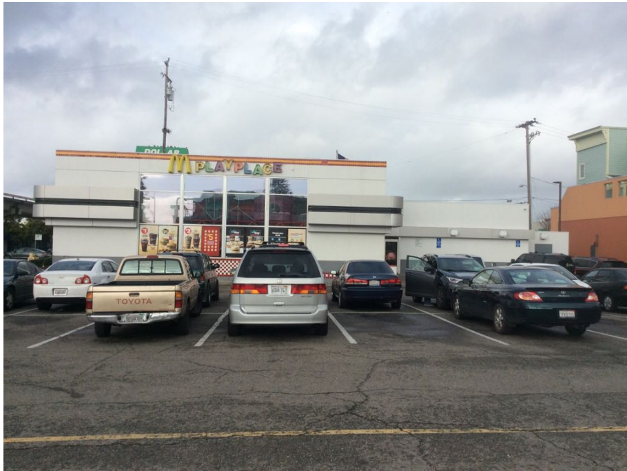
Photo – 9 – Non Drive-Thru Side of Building
