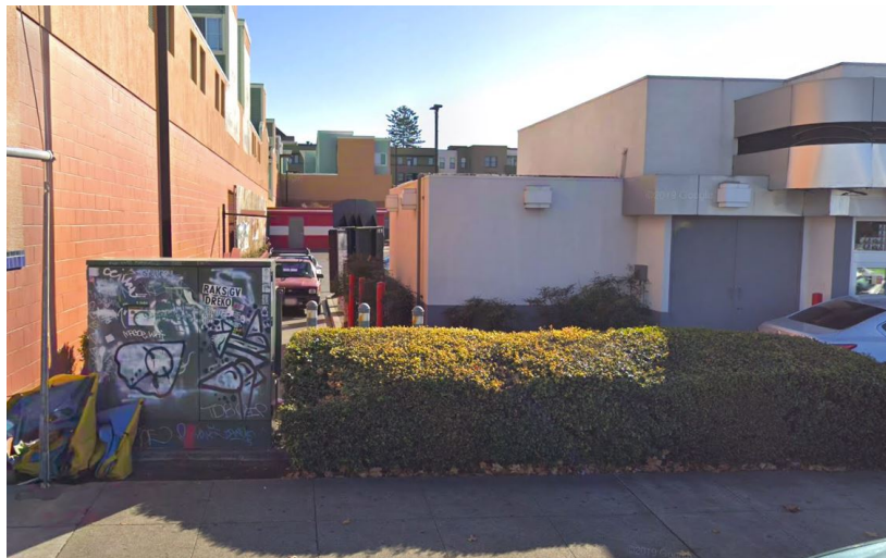
Photo – 11 – Rear Elevation Side of Building at Exit
