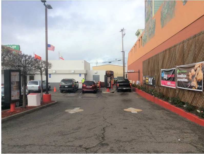
Photo – 10 – Rear Elevation Side of Building @ Entry
