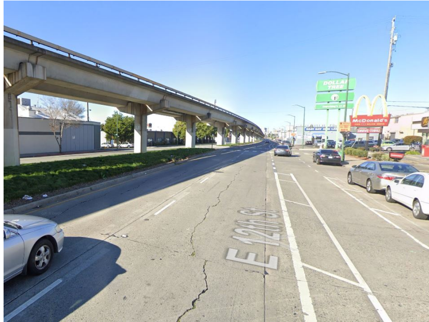
Photo -1- E 12th going North West
