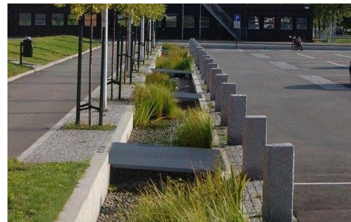
BIORETENTION BASIN w/ METAL GRATE
