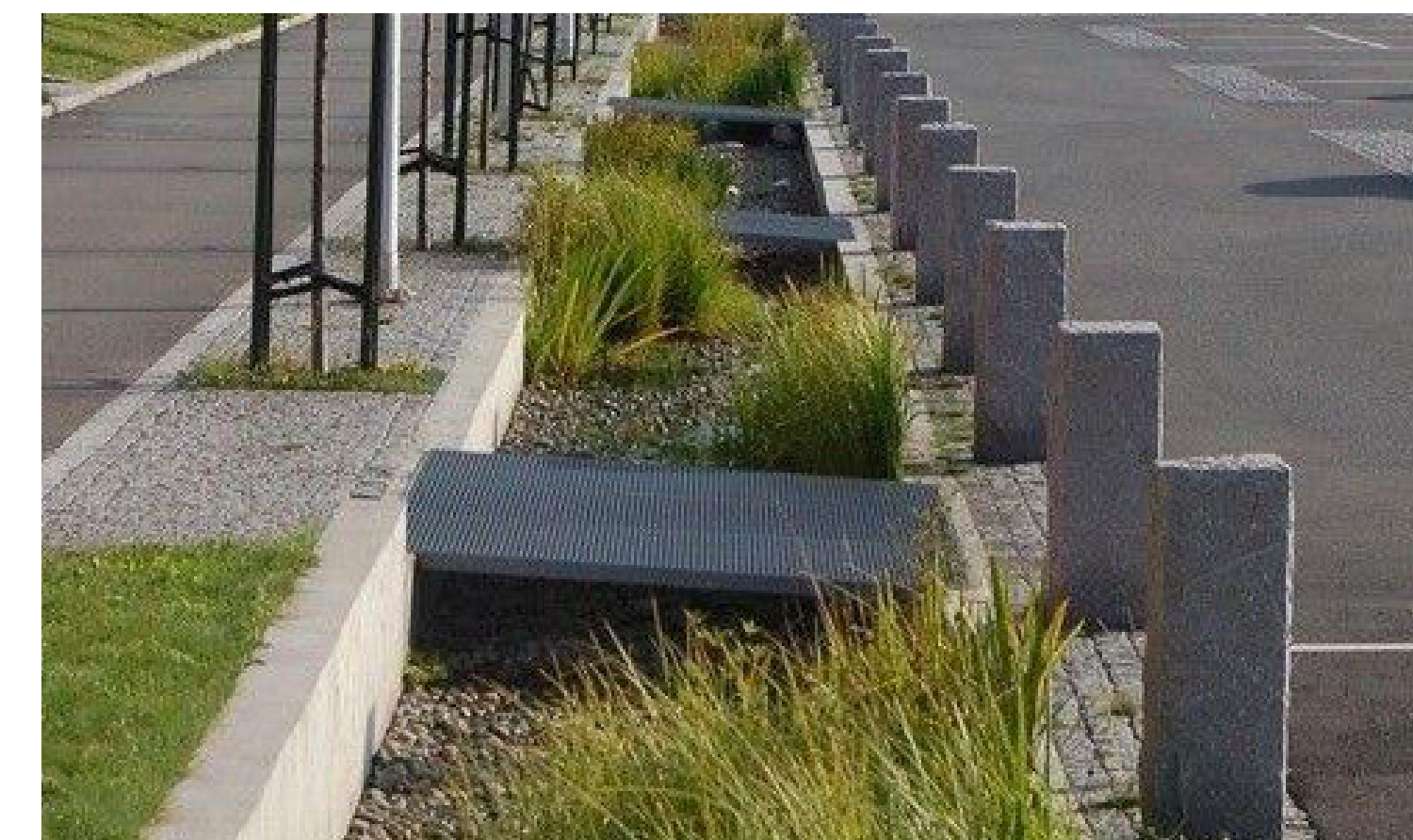
BIORETENTION BASIN w/ METAL GRATE
