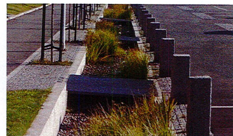
BIORETENTION BASIN w/ METAL GRATE
