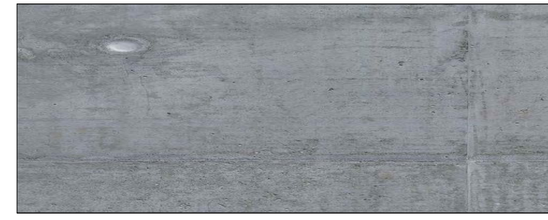
C1 CONCRETE - EXPOSED
