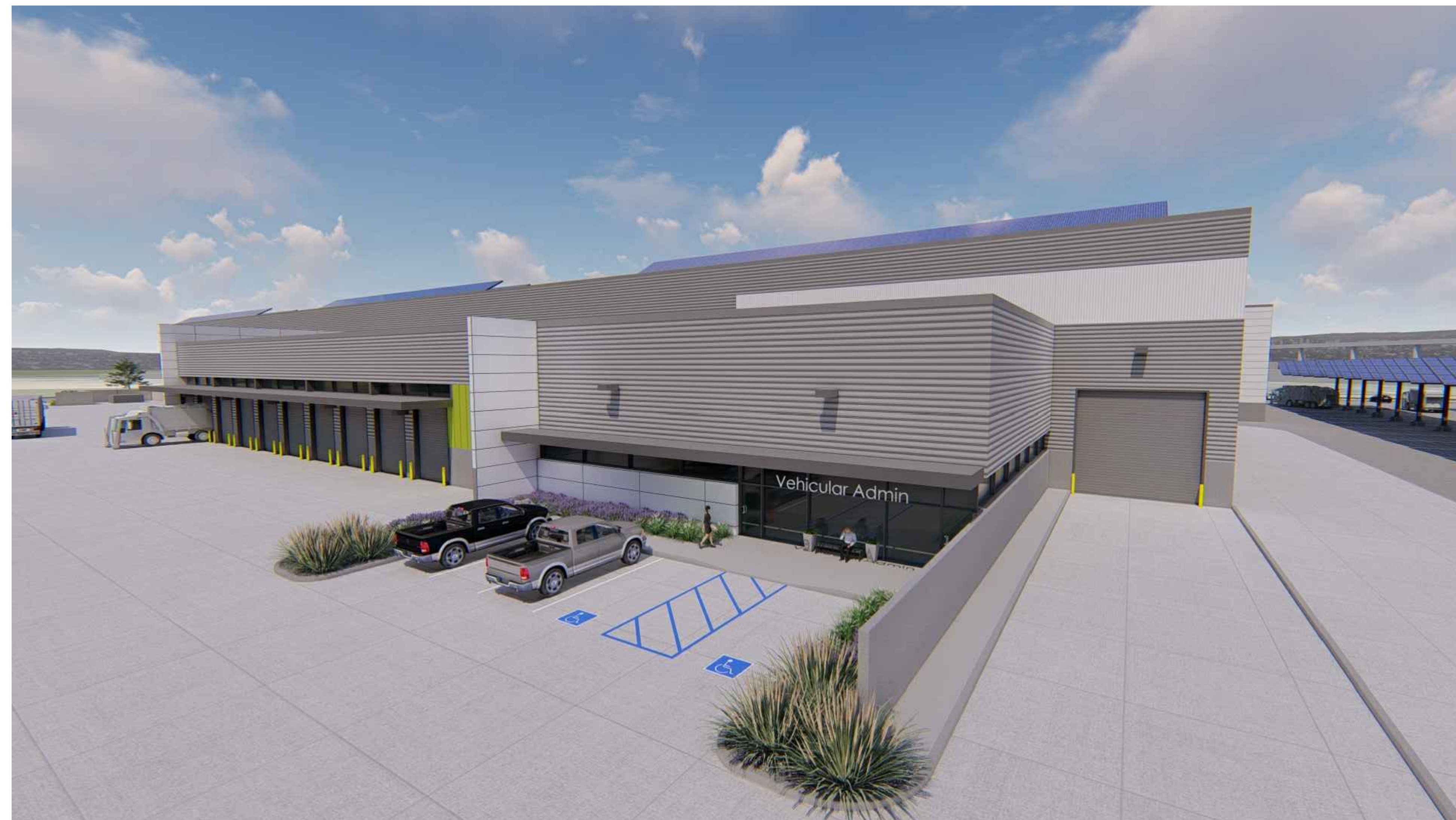
4. View from South East Corner of Building at Maintenance Shop
