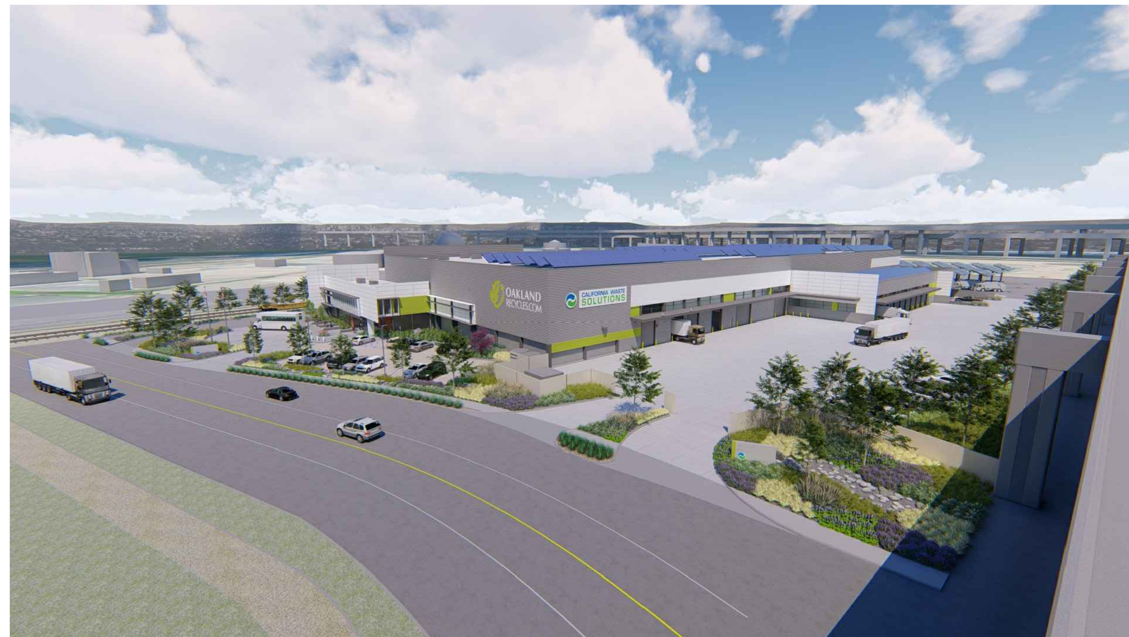
2. Elevated View South West Corner of Property
