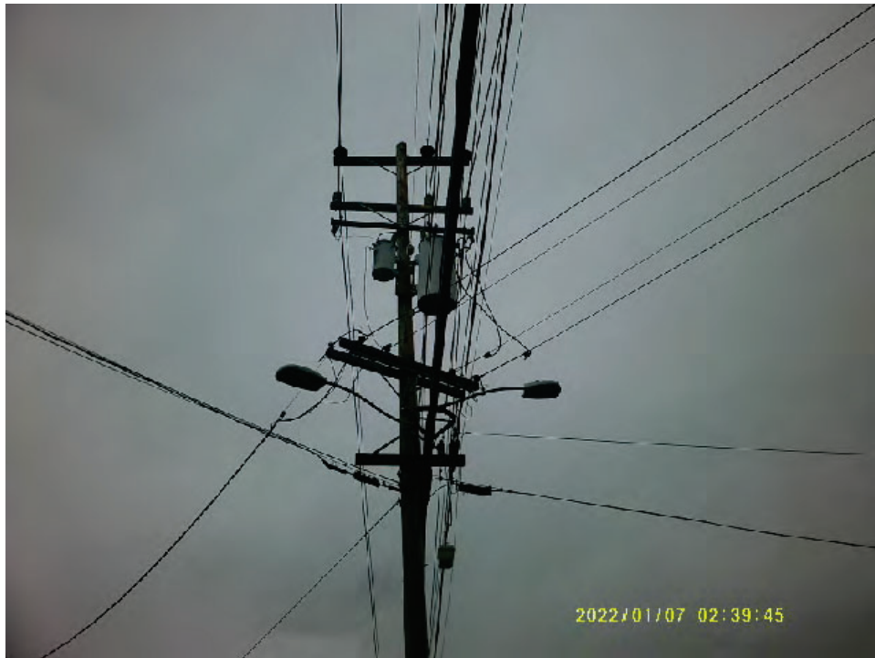
16. Pole-mounted transformers
