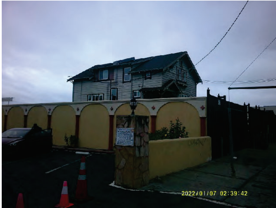
23. Adjacent northwest - residence with auto repair
