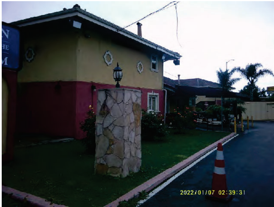
3. Northwest side of subject property main building
