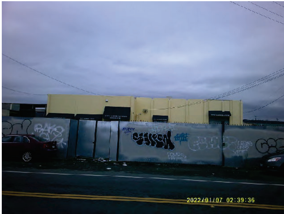
24. Adjacent northeast - plaster casting warehouse across Coliseum Way
