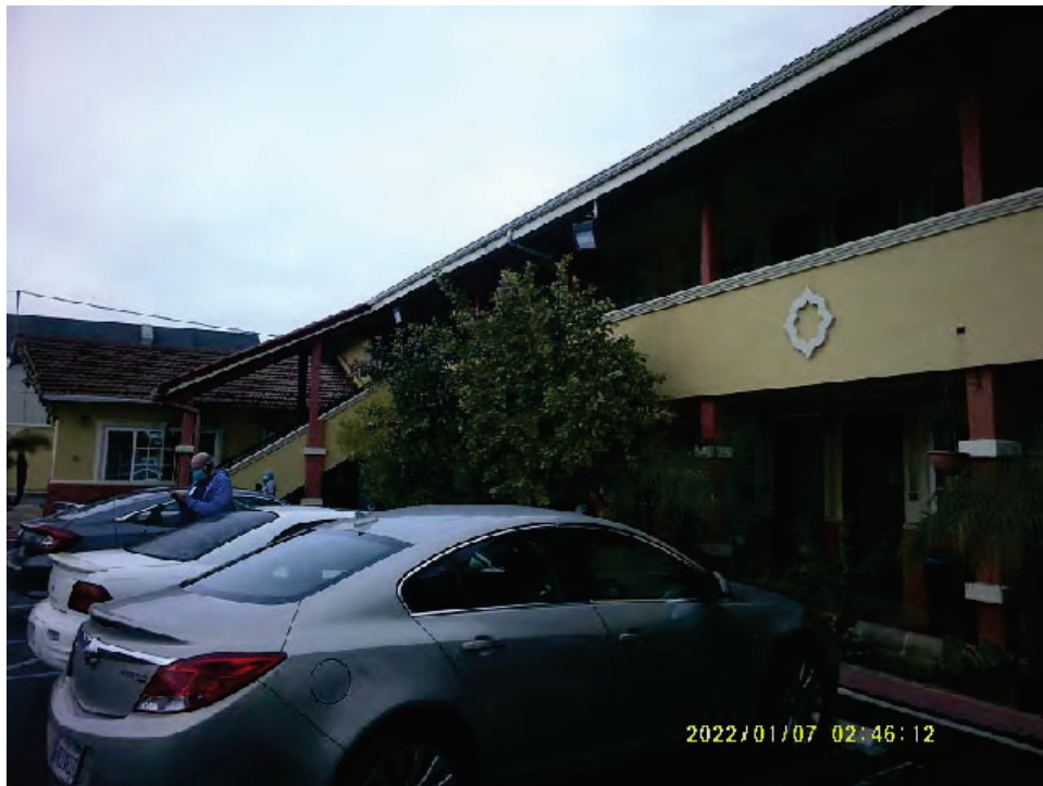
2. Southwest side of subject property main building
