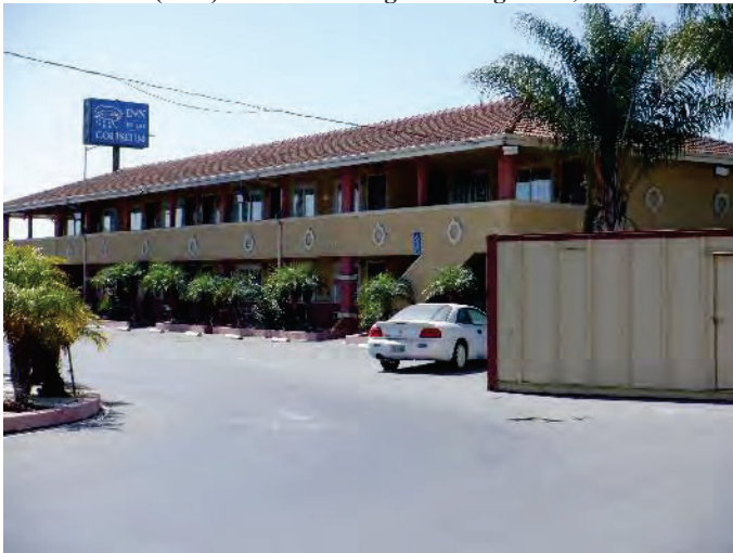
Photograph 4: West building. Camera facing southwest. August 31, 2022.
