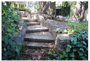
Figure 165. Staircase paved with Carnegie bricks, flanked by masonry retaining walls with ceramic pots.
