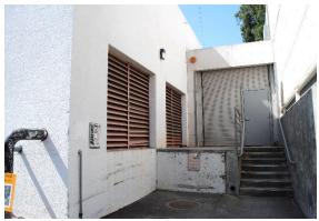
Figure 122. Two large vented openings at the north end of the west façade of Shaklee Building (left), looking south. A hyphen addition attaches to Barclay Simpson Sculpture Studio (right).
