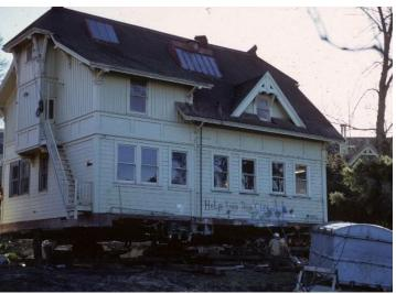
Figure 24. West and north facades of the Carriage House raised up on temporary foundation for relocation, 1973.
