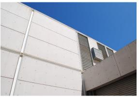
Figure 142. Steel grid structure with fiberreinforced concrete boards fastened by screws on the east façade, looking west. Metal vents are visible above the central hyphen volume.
