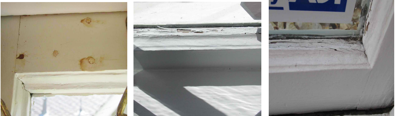
Some wood is dry-rotten but most damage is the result of aging putty, sun exposure and water seepage.
