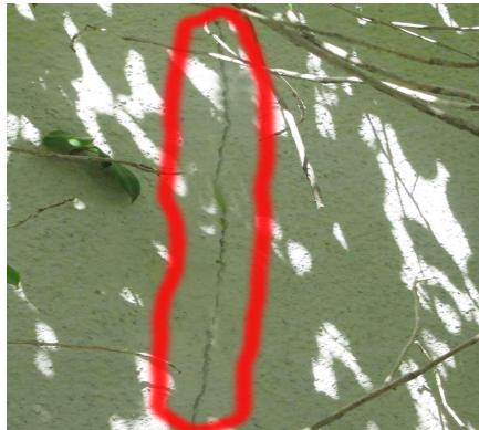
Cracks in stucco reappear on a regular basis and need to be addressed to prevent damage.
