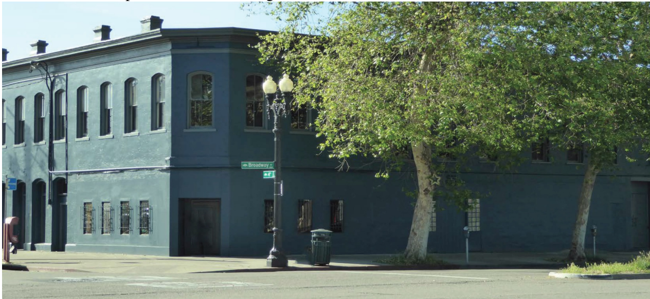
2018 – Google Maps – Showing Vacant Building at Time of Purchase by Developer
