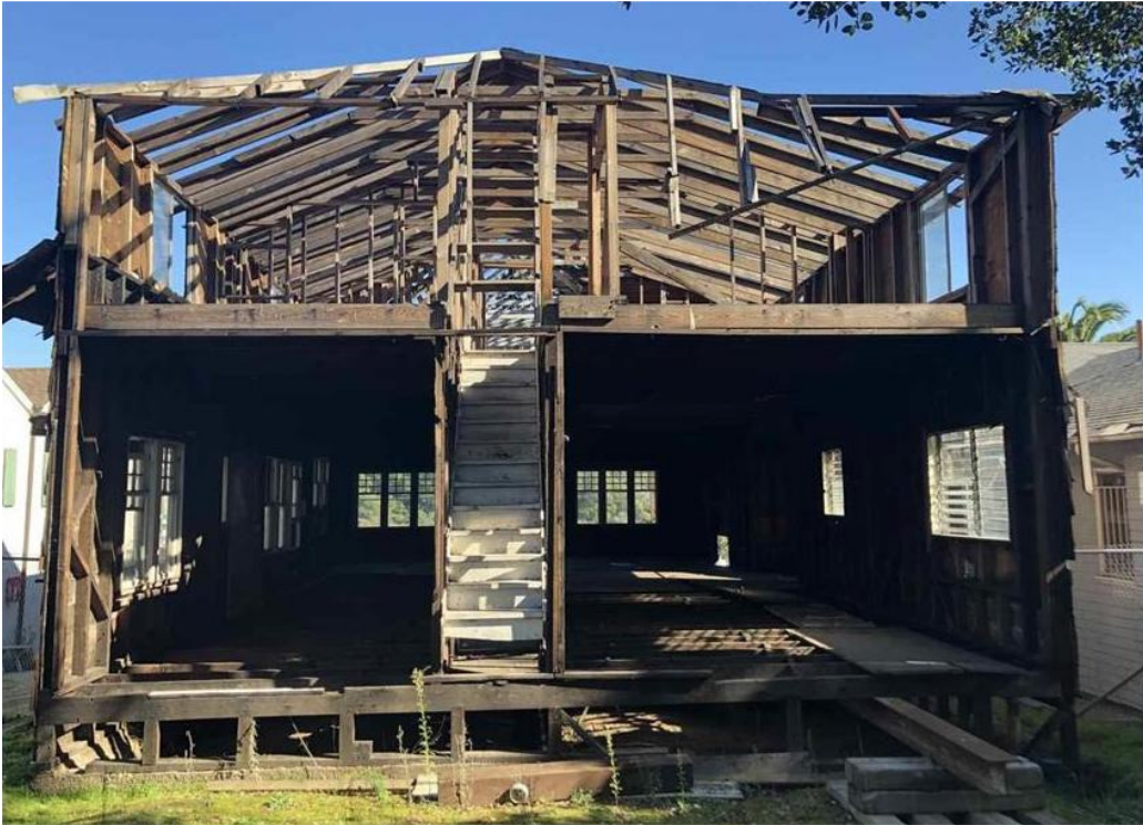
Rear of building from backyard
