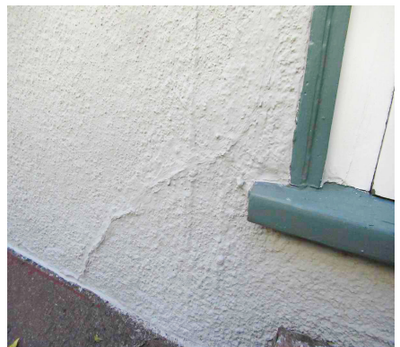
Cracks in the stucco walls are often hidden by the mature landscaping.
