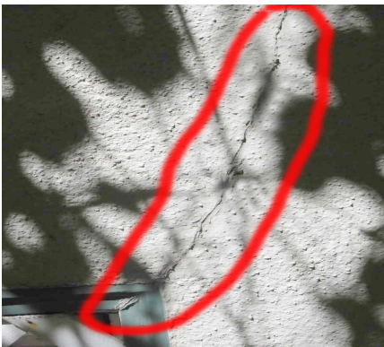
Cracks in the stucco walls are often hidden by the mature landscaping.
