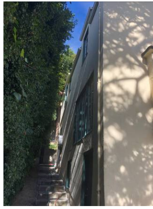
Left Side of the House
