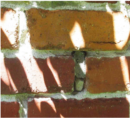
Bricks on pillars, porch and chimney need to be sealed and, in some cases, re-pointed.
