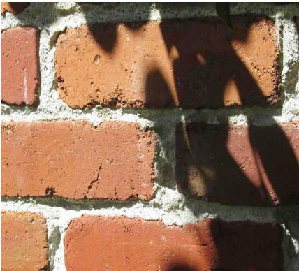
Bricks on pillars, porch and chimney need to be sealed and, in some cases, re-pointed.
