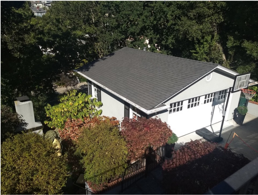
Figure 7. Garage, view facing northeast.
