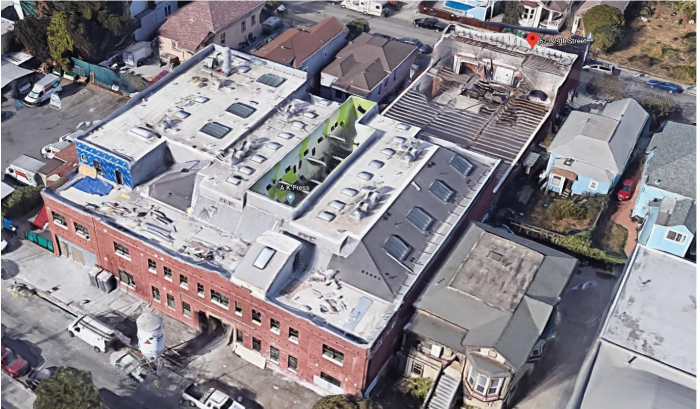
Aerial View of 23 rd Street and 24 th Street combined buildings.
