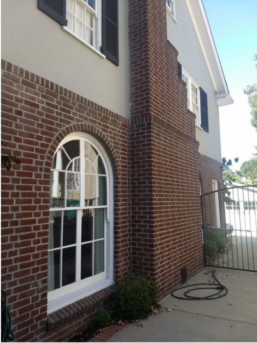
Figure 2. 676 Longridge Road, east side elevation, view facing northwest.
