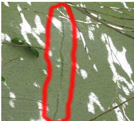
Cracks in the stucco walls are often hidden by the mature landscaping.
