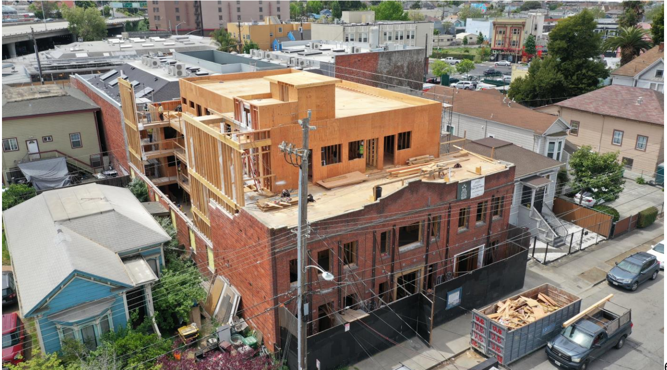
24 th Street interior addition progress.
