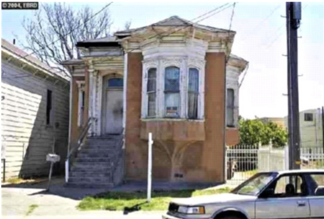
(2004) The Martin House covered in stucco and in disrepair.
