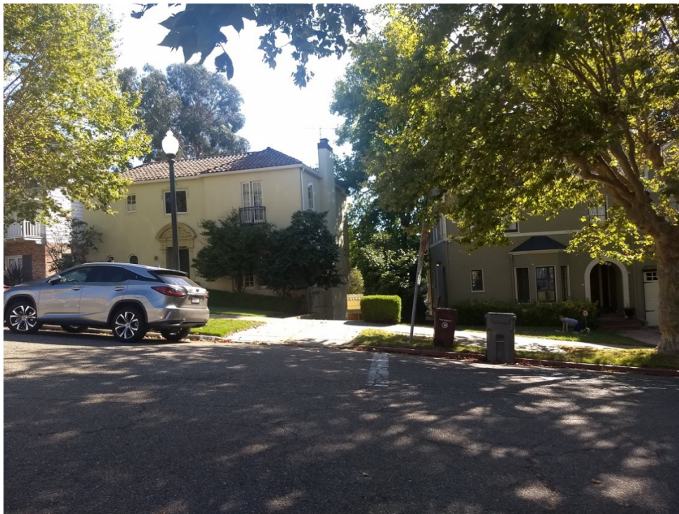
Figure 10. South side of Longridge Road, across the street from the subject property, view facing southeast.
