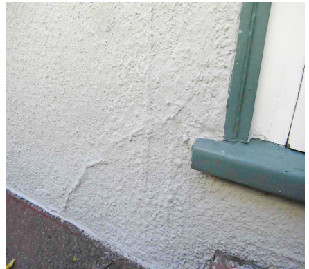
Cracks in stucco reappear on a regular basis and need to be addressed to prevent damage.
