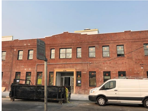
674 23rd St (south) facade, camera facing north
