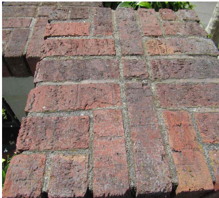
Bricks on pillars, porch and chimney need to be sealed and, in some cases, re-pointed.
