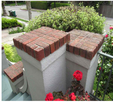
Periodic reapplication of brick weather sealer will prevent water seepage and dry rot.
