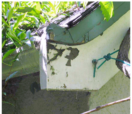
Cracks in stucco reappear on a regular basis and need to be addressed to prevent damage.
