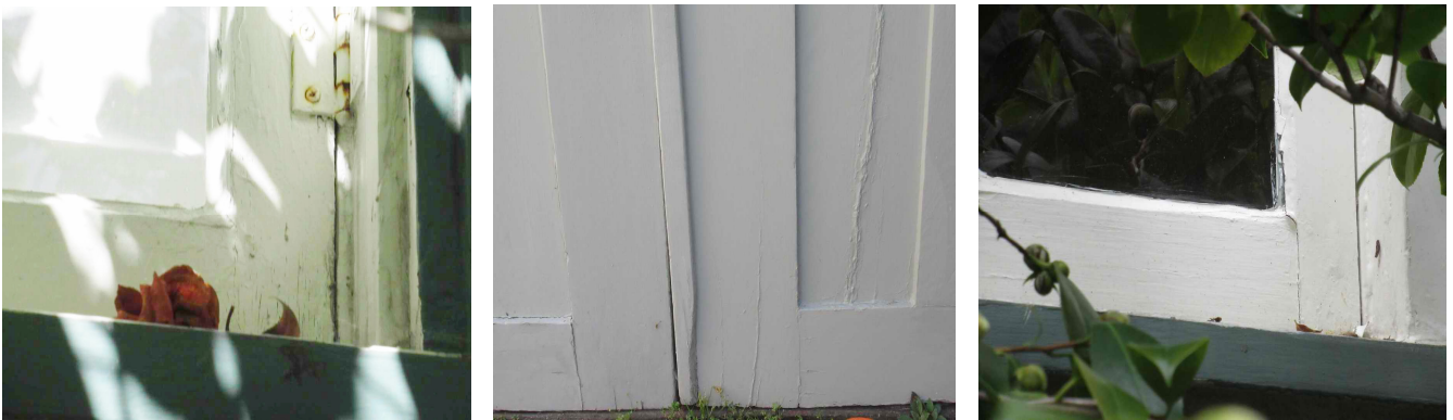
Some wood is dry-rotten but most damage is the result of aging putty, sun exposure and water seepage.
