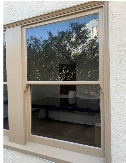
Typical off-street window
