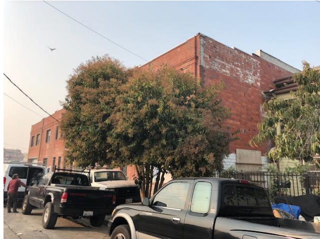
674 23rd St southeast corner, camera facing
