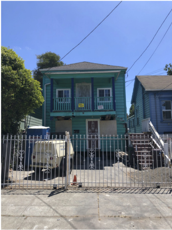
Front of house, January 2019
