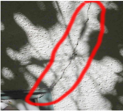
Cracks in stucco reappear on a regular basis and need to be addressed to prevent damage.
