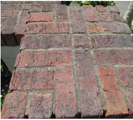
Periodic reapplication of brick weather sealer will prevent water seepage and dry rot.
