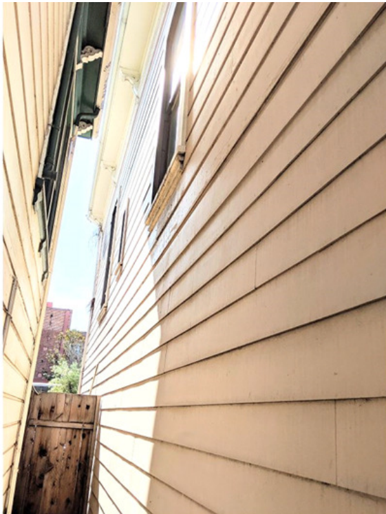
Left side (alley) view
