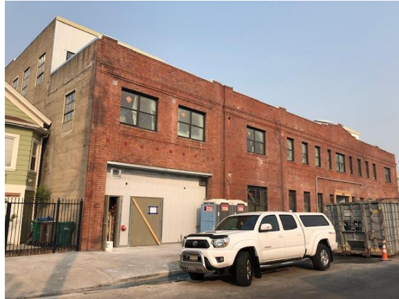
674 23 rd Street (South Façade)
