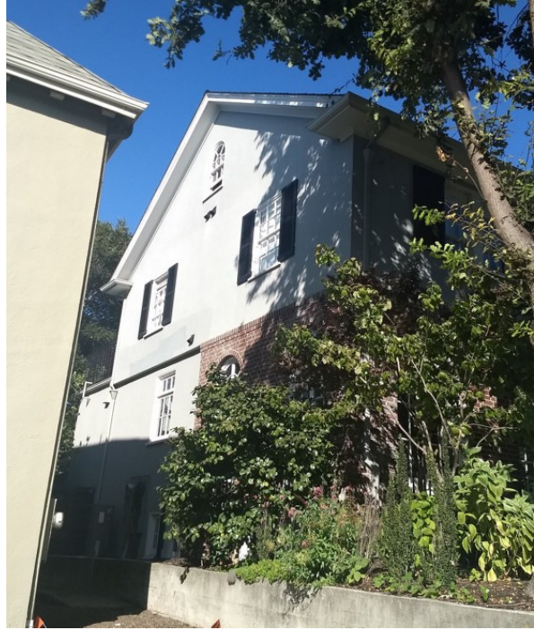
Figure 3. 676 Longridge Road, west side elevation, view facing northeast.
