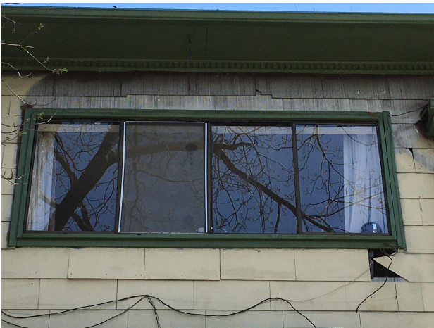
detail of aluminum windows on right side
