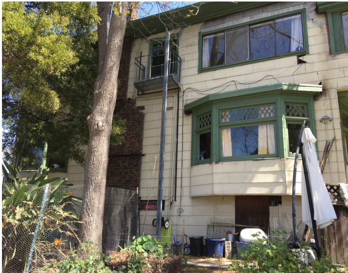
Right side of house – asbestos siding, original vs aluminum sash
