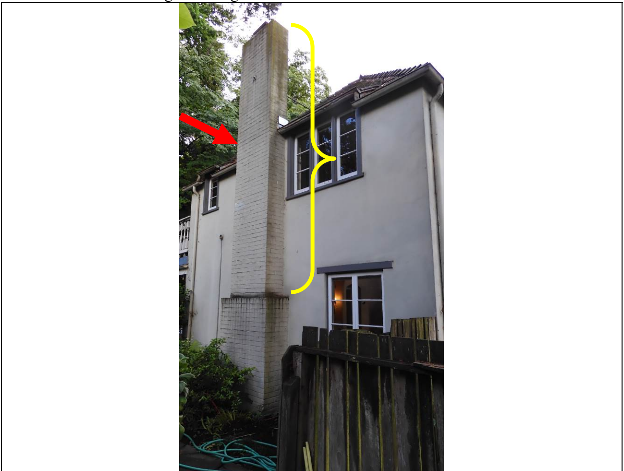
Work Item #5 - Photo 1 Replace upper masonry chimney stack to make seismic safe (yellow bracket) (visually “like for like”). Lower fire box remains. Red arrow depicts a large horizontal crack. Chimney leaning towards roof.
