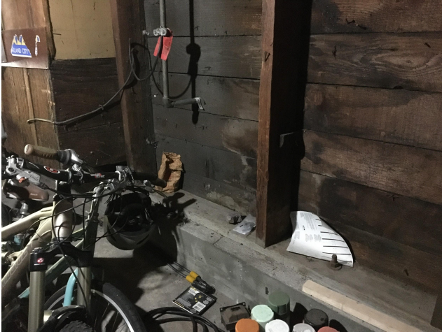
right side foundation wall
