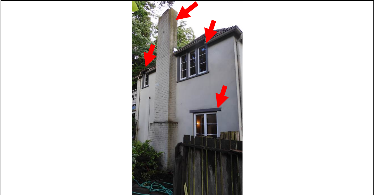
Work Item #8 - Photo 1- Paint windows and waterproof as needed. Clean and paint chimney and chimney with structural attachments.
