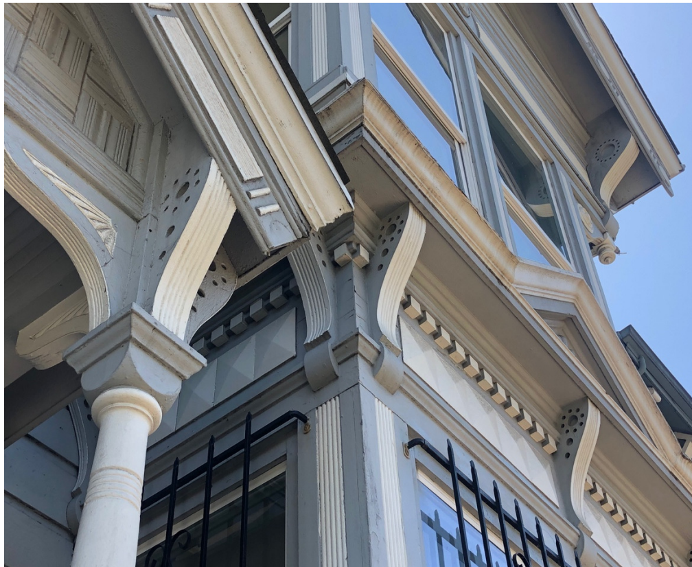
Geometric perforated brackets, small under 1 st story eaves, large under the roof line; checkerboard and wing motifs in porch gable (at left)
