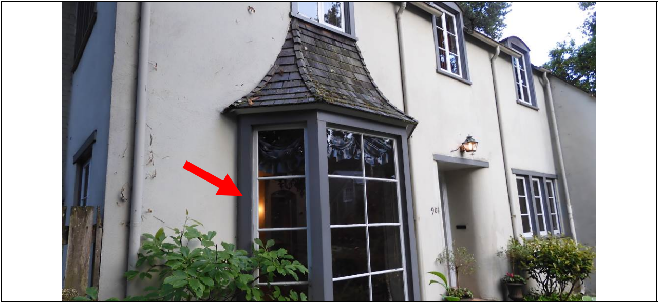
Work Item #5 - Photo 2 Bay window maintenance.
