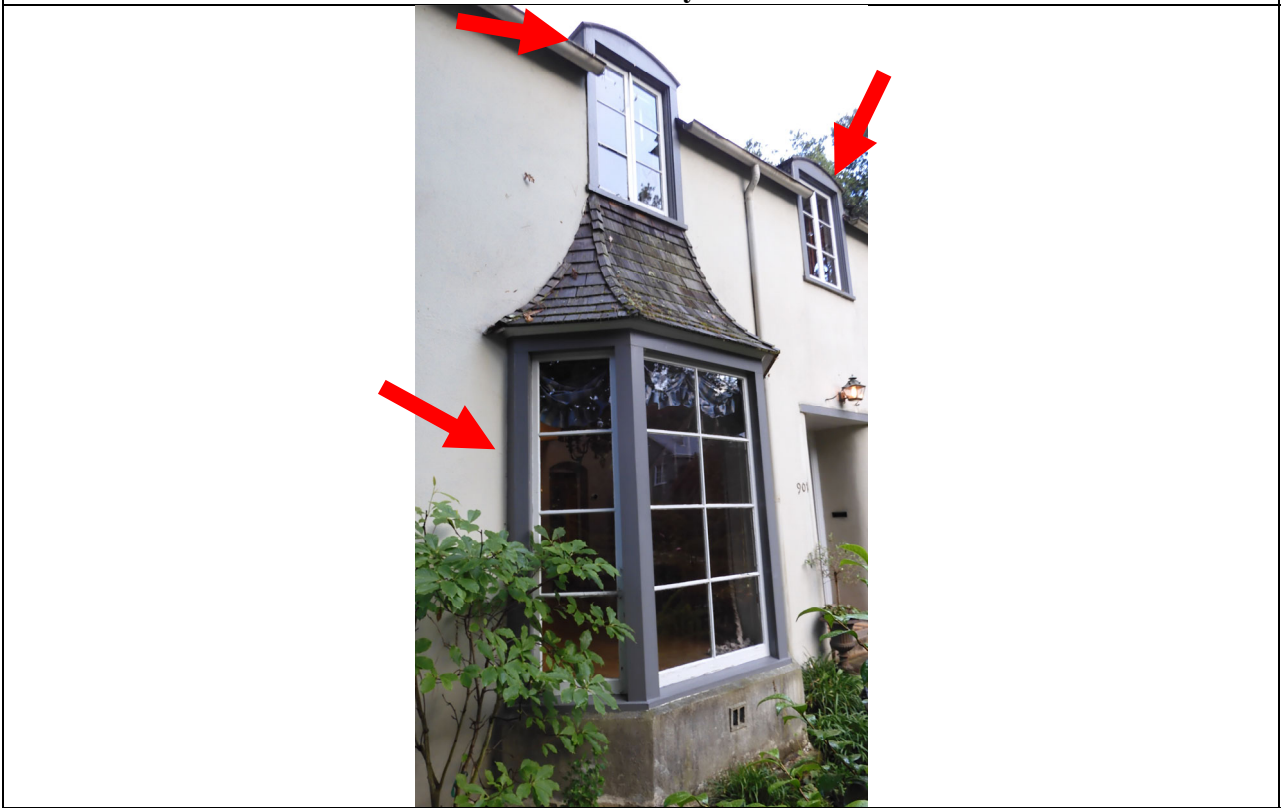
Work Item #5 - Photo 3 Bay window and upper gable maintenance.
