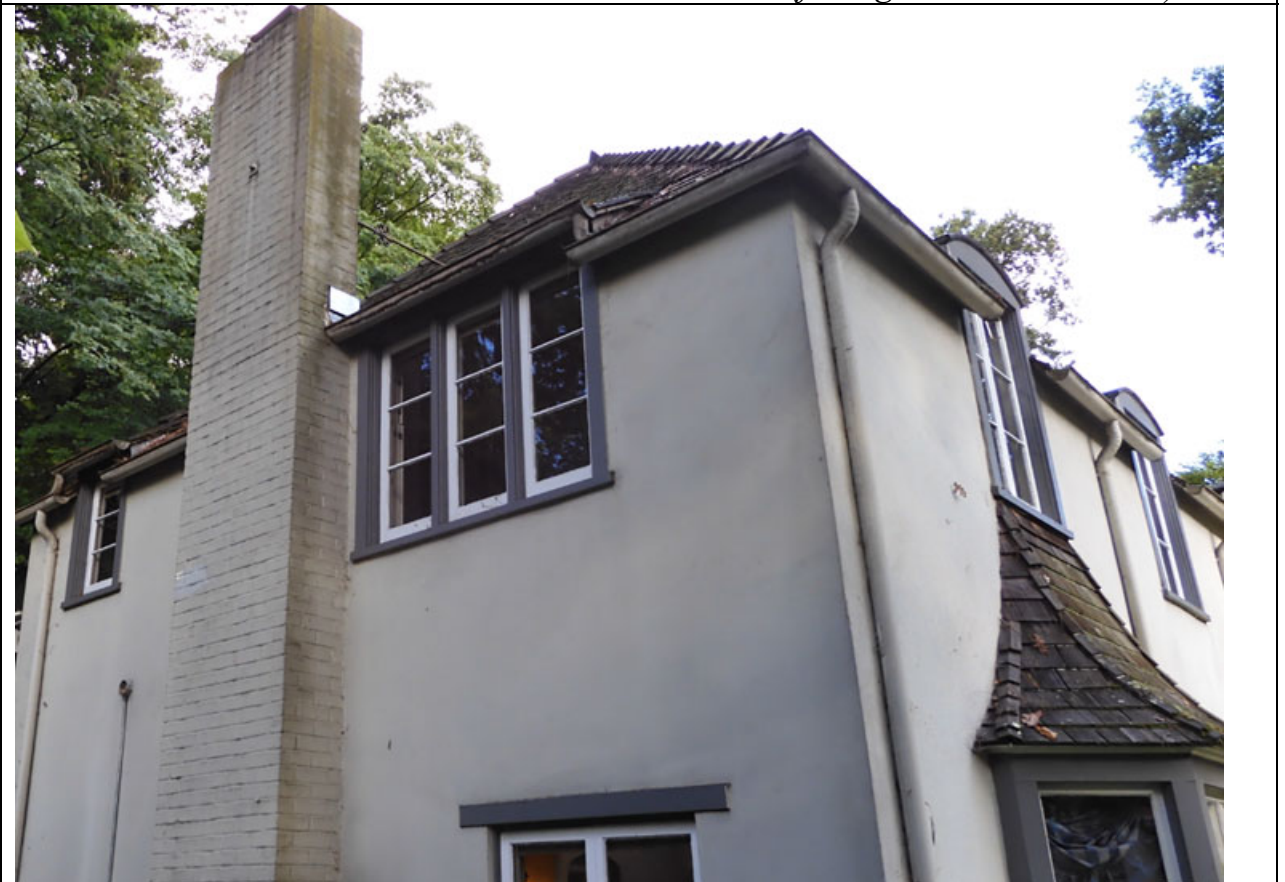
Photo B Side Southern Elevation House View (facing Warren Hook Park)
