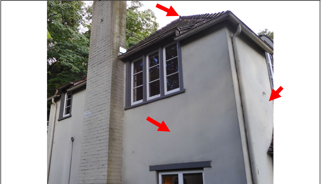
Work Item #10 – Photo 1- Repair and paint stucco and waterproof as needed. Clean and repair wood single roof as needed.
