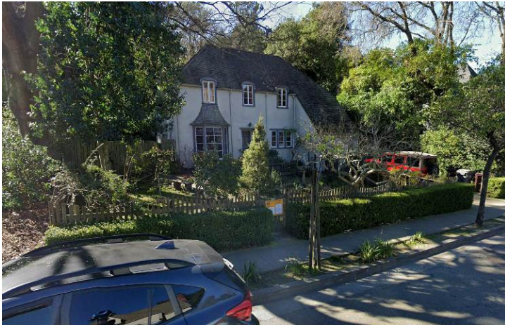
View looking northwest at 901 Trestle Glen
