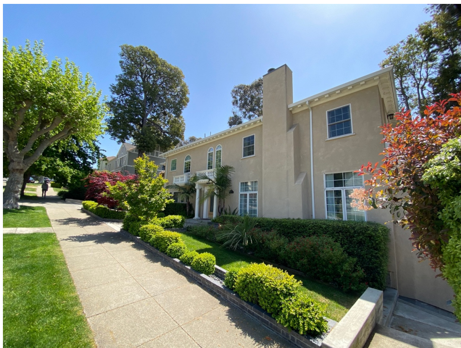
671 Longridge Road, Northwest Façade, 2021
