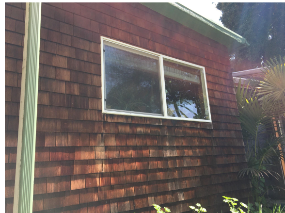
detail of downstairs addition window
