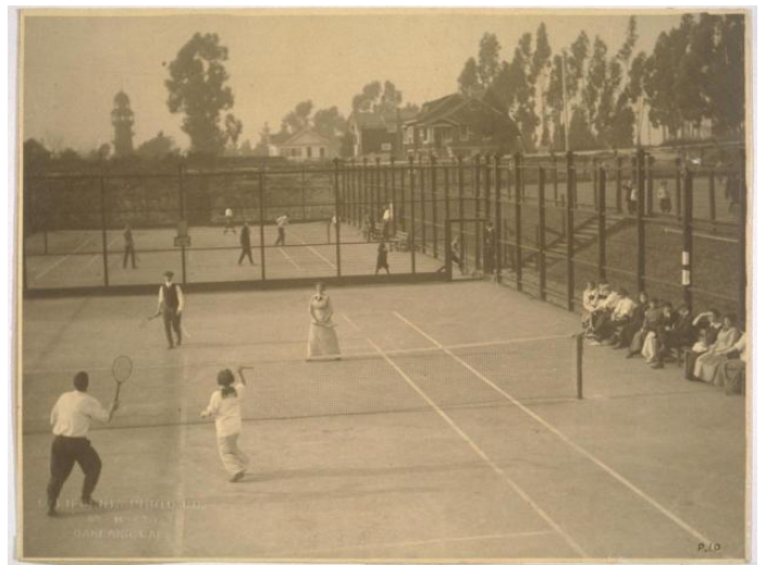
Tennis Courts at Bella Vista Park, notice the Arbor Villa estate Observation Tower located in the upper left
