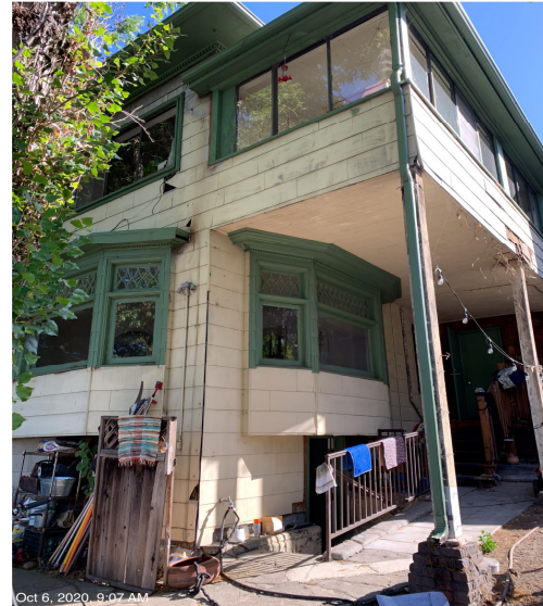
Rear – stabilize upper sunporch as part of foundation work
