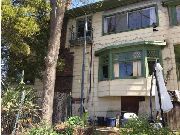
right side of home, aluminum windows above bay
