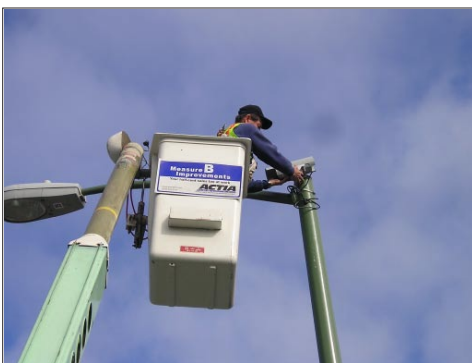
City crews install video detection camera on street light.
