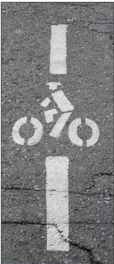
Bicycle detector pavement marking
