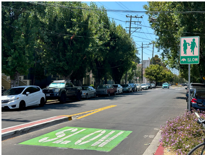
Slow street features at 8th St and Mandela Pkwy, including hardened centerline, “slow” pavement marking and “slow st” sign
