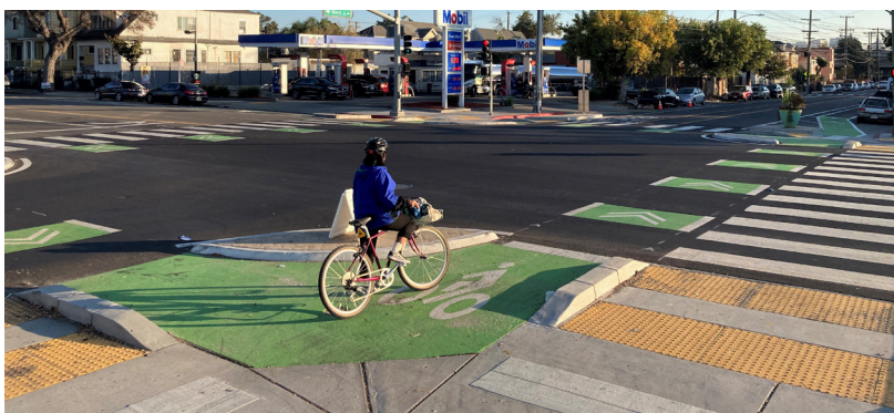
Protected intersection at West St and 27th St that will be swept by the Multihog
