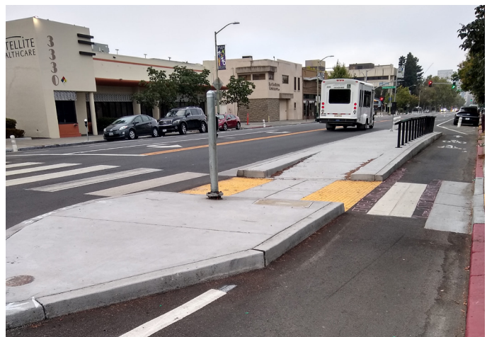
Bus boarding island adjacent to a separated bike lane, continuing from and to a buffered bike lane, and a pedestrian safety island.
