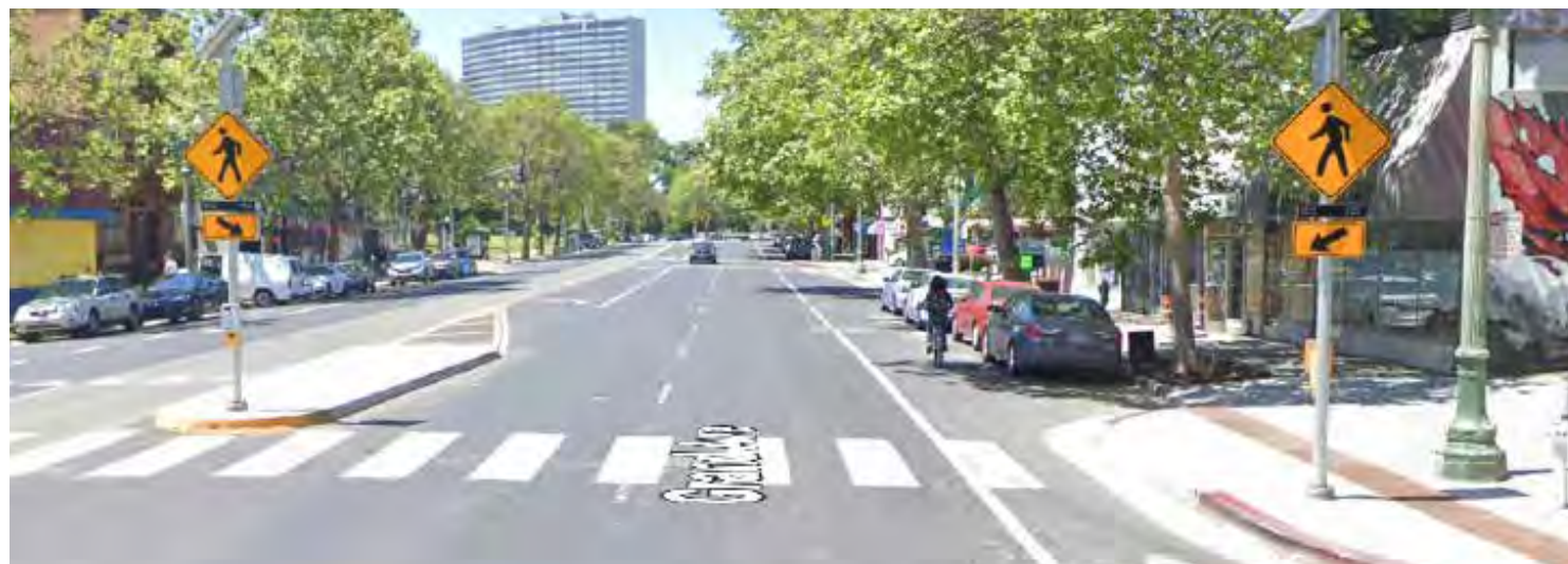
RRFB at Grand Avenue and Ellita Avenue in Oakland
