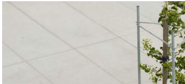
CIP CONCRETE, SAWCUT, SANDBLAST
