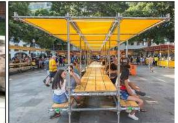
GALVANIZED PIPE SCAFFOLDING + TIMBER BENCH
