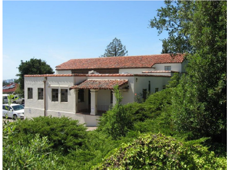
Figure 4.06: Existing Building 0 from South
