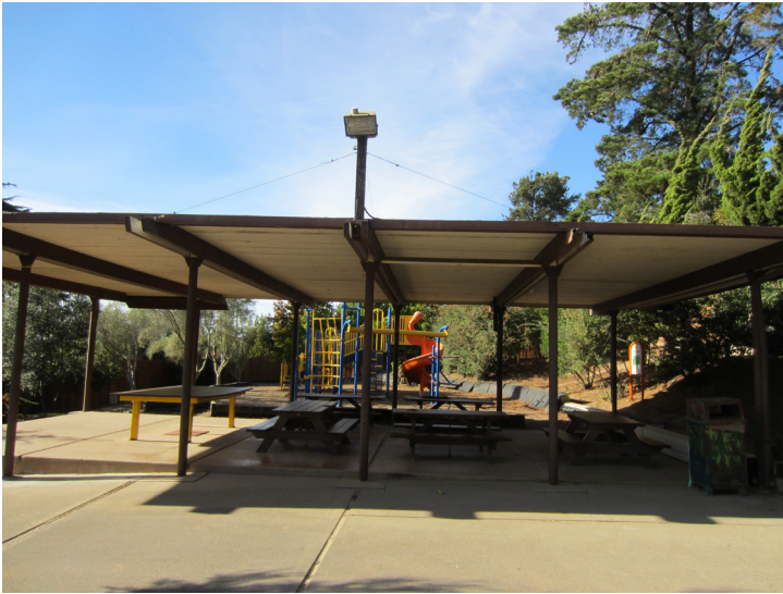
Figure 4.09: Existing Canopy and Play Structure
