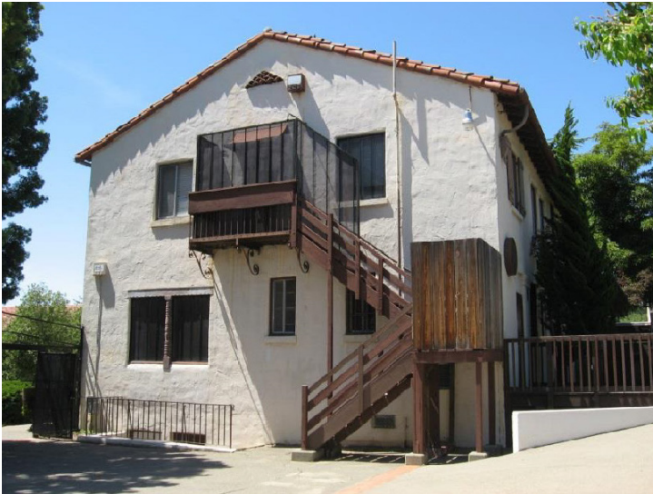
Figure 4.07: Existing Building 1 from South
