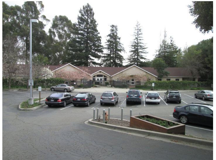
Figure 4.12: Existing Parking Lot C and Building 9
