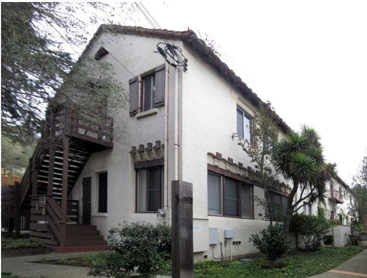
Figure 4.11: Existing Building 2 from Northwest
