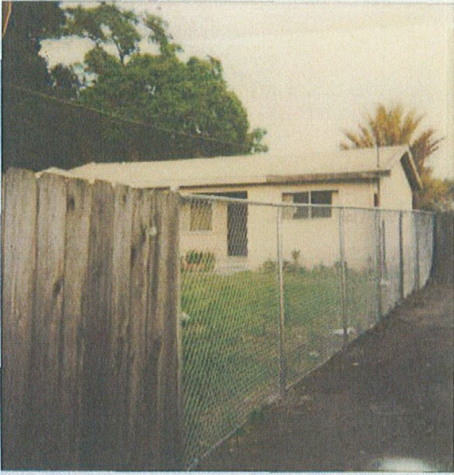
5-15-01 1354-81 st Ave Back-Done L-Side Fencing
