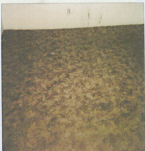
5-9 1354 81 st Ave APT-13 Done Bedroom / 10 th side
