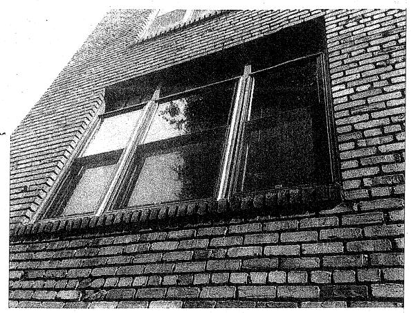
Evidence of work not complete as of 3/11/17 (white caulking substance)
