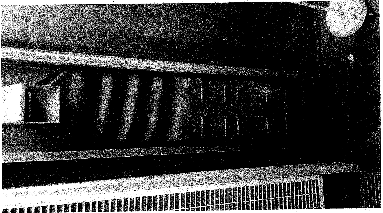
Exhibit 3, picture of heater taken 4/11/2018, removal of parts.
