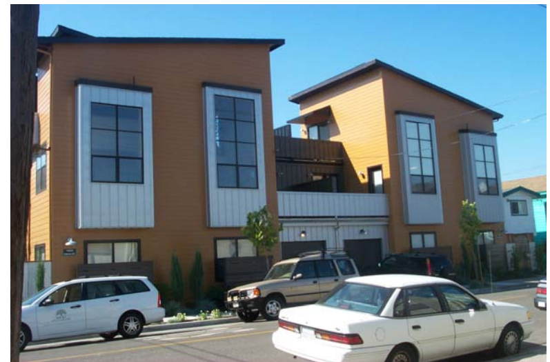
Guideline 3.1: The private usable open space above the garages of this duplex is convenient to both units and incorporated into the design of the building.
