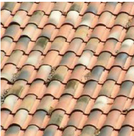
CLAY TILE ROOF
