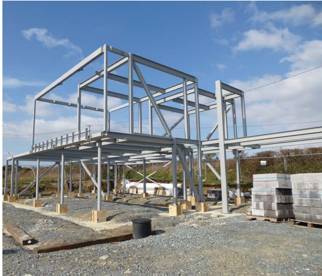
BUILD STEEL SKELETON
