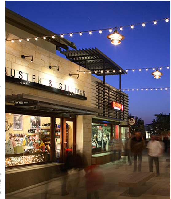
Lighting and Signage
