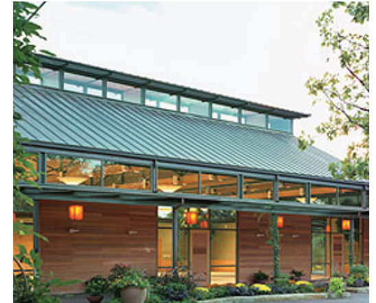
Clerestory windows and natural lighting
