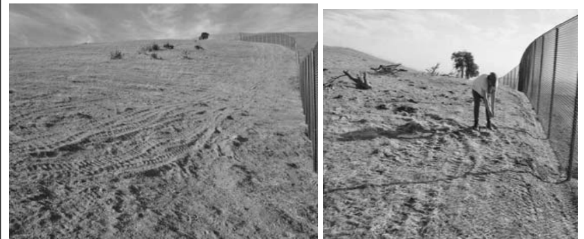
Figure 2. Knowland Park hillside immediately above Zoo with approximately 530 linear feet (estimated .41 acres) of unpermitted damage to protected grassland from construction equipment. Extensive soil-tear on both development and public sides of perimeter fence. Use of equipment here (Site Areas C–D) is prohibited by both CDFW and City permits. Complaint sections 1a–e, h, 2a, c, d.
