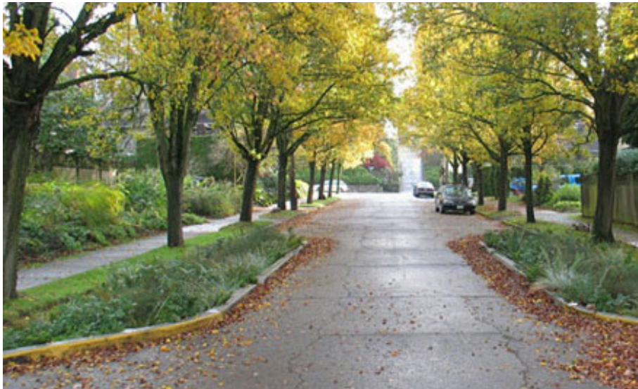
Integrated Stormwater Treatment - "Rain Gardens"
