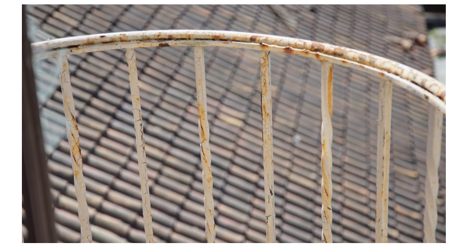
MTL-1 RESTORED METAL RAILINGS
