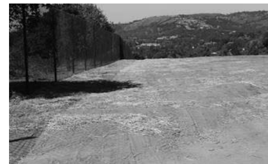
Figure 7. Unauthorized damage by prohibited equipment to protected native grassland along east-facing perimeter fence in public parkland outside the development footprint (Site Areas E2–F). Approximately 450 linear feet x 25' = estimated .26 acres. Complaint sections 1a–d, f, h; 2a, c, d.
