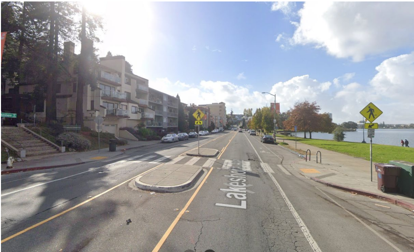
Looking south at Cleveland Cascade
