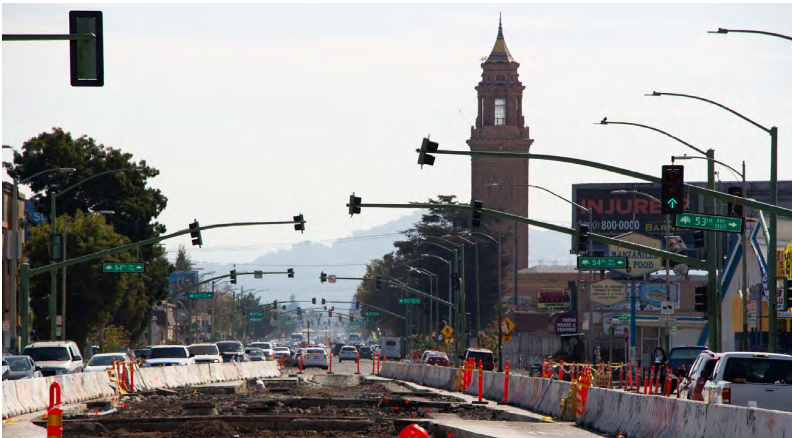
International Blvd and 53rd Street Under Construction, 2019 UC Berkeley Transportation Studio.
