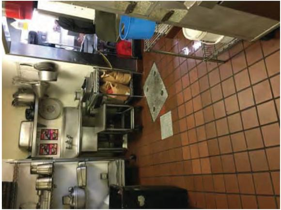
Photo 3. Kitchen at Merritt Bakery, grease trap can be seen on the floor on the right side of the frame, 500 Lake Park Avenue, Oakland, California
