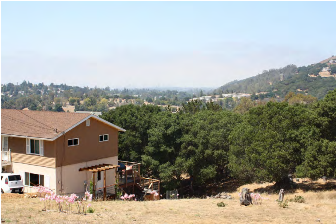
Existing view from Briarcliff Road looking northwest (VP E)
