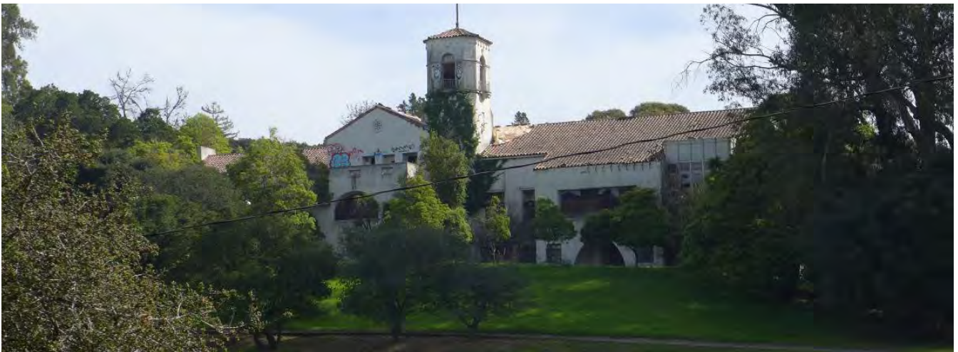
West elevation viewed from former golf course, 2016
