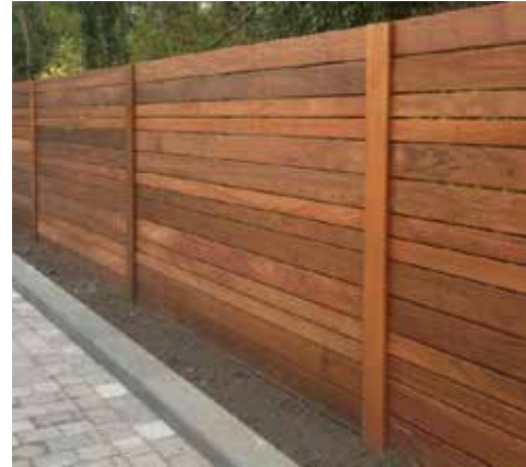
WOOD FENCE - HORIZONTAL BOARD, 6' HEIGHT. MATERIALS PER OAK KNOLL DESIGN GUIDELINES MAXIMUM 12" STEPDOWN BETWEEN PANELS.
