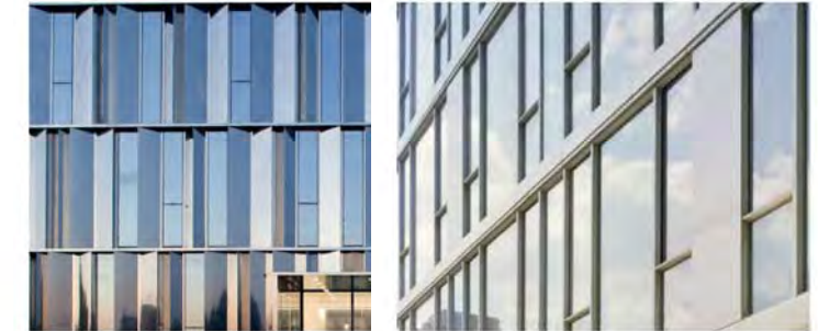
Window Wall System (Kawneer, Equal or better)
