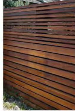
WOOD FENCE - HORIZONTAL BOARD, 6' HEIGHT. MATERIALS PER OAK KNOLL DESIGN GUIDELINES
