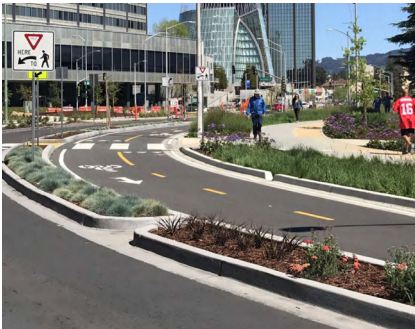
Harrison Street Bioswales (Source: Oakland GSI Plan)
