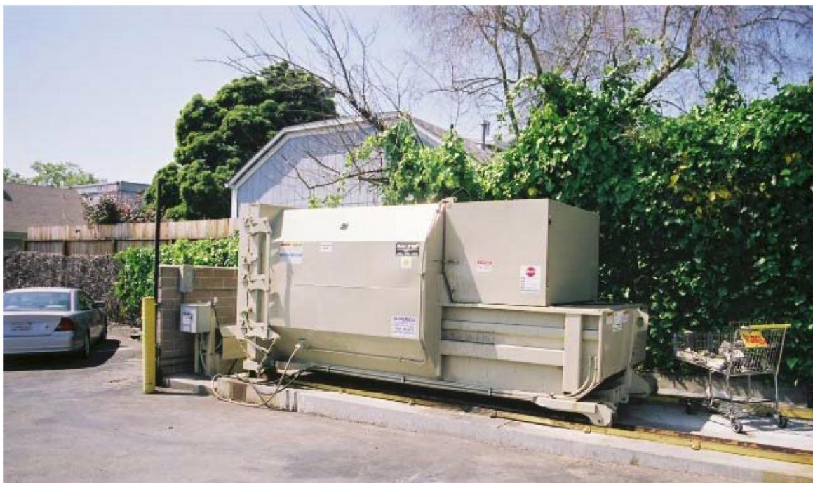
2. Existing Trash Compactor adjacent to Residential Property Boundary
