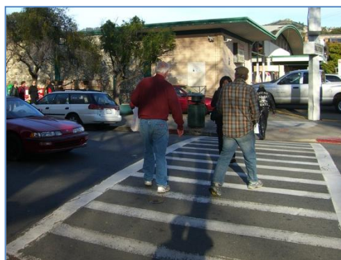
High-Visibility Crosswalk across College Avenue at 63 rd Street
