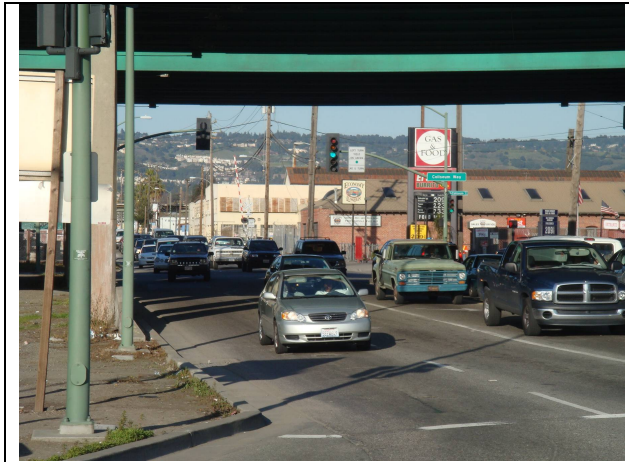
Roadway environment on Fruitvale Avenue as it passes under I-880
