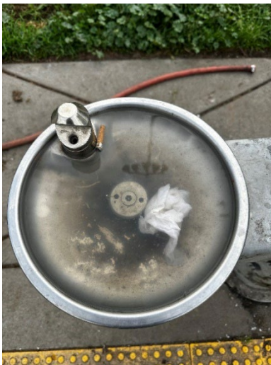
Nonfunctioning and clogged water fountain
