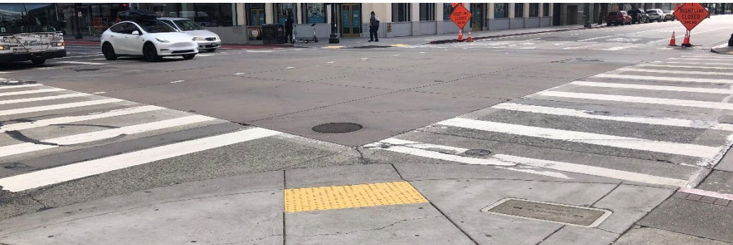
Curb ramp design that don't facilitate safe, accessible crossings
