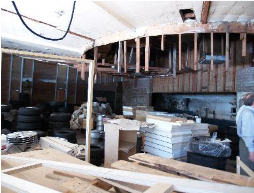
Figure 8. Interior, looking toward former counter and open kitchen, Page & Turnbull, July 2007
