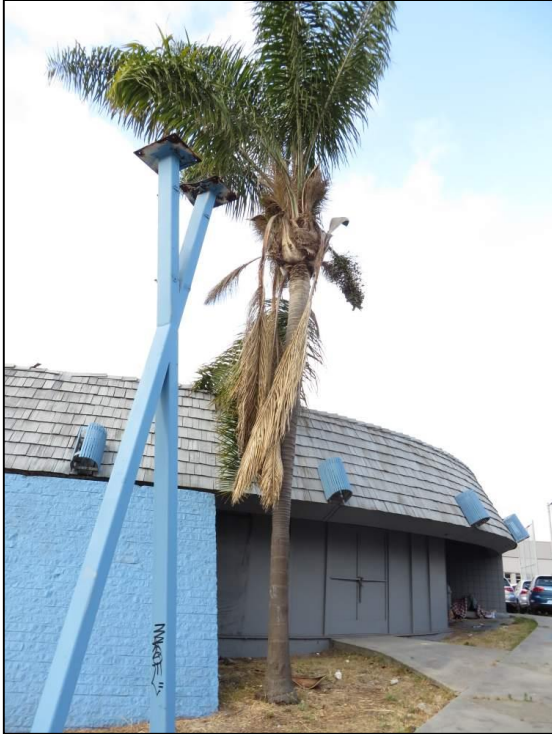
Photo 5 – Queen palm #186 was growing 1 foot away from the building and had two dead fronds hanging.
